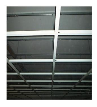
The AAF inverted T-bar ceiling grid is a 55 mm wide ceiling grid system designed to accommodate individual filter modules, blank panels and lay-in-light fixtures in ISO Class 5 to ISO Class 8 cleanrooms. For ISO Class 5 applications, the entire cleanroom ceiling is composed of AstroCel TM Filter Hoods, AstroFan FFU filters and teardrop light fixtures.
