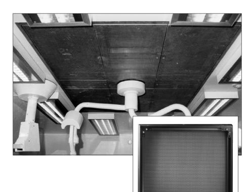
The CR II module is suitable for installing exchangeable particulate filters such as the AAF-AstroCel II.
